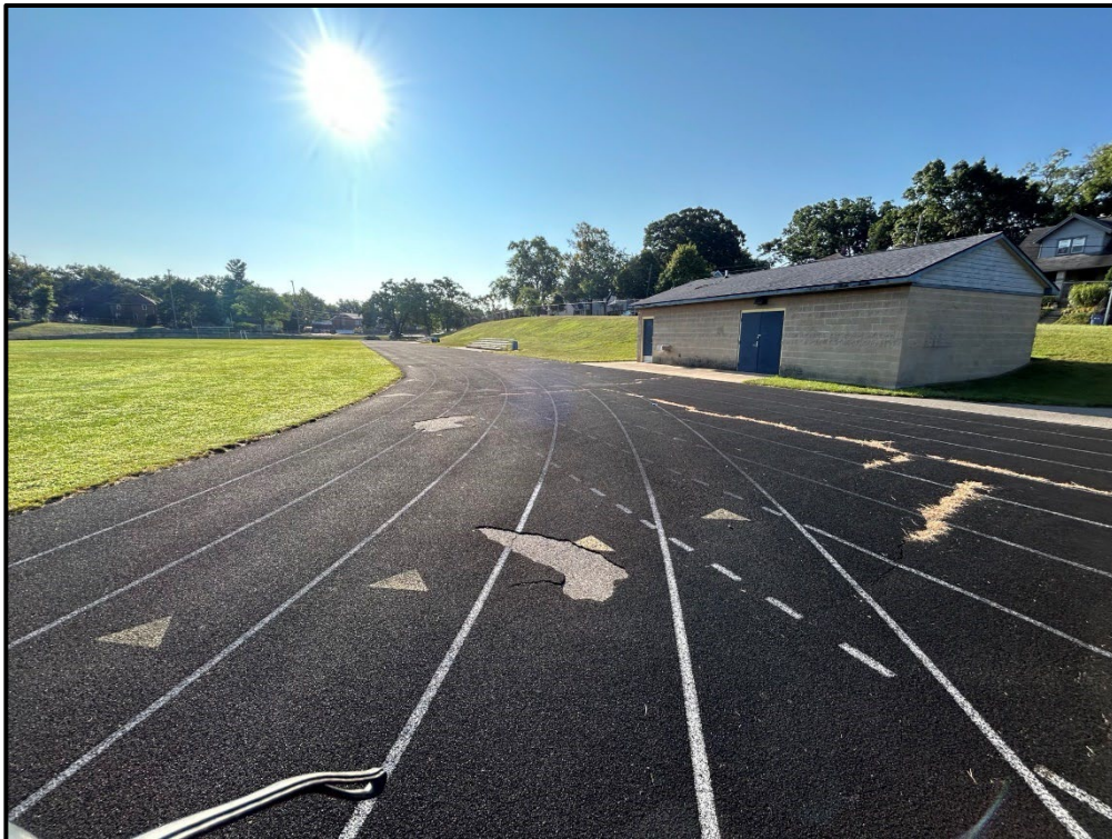
Briggs Field, track surface near the southwest corner, looking east
