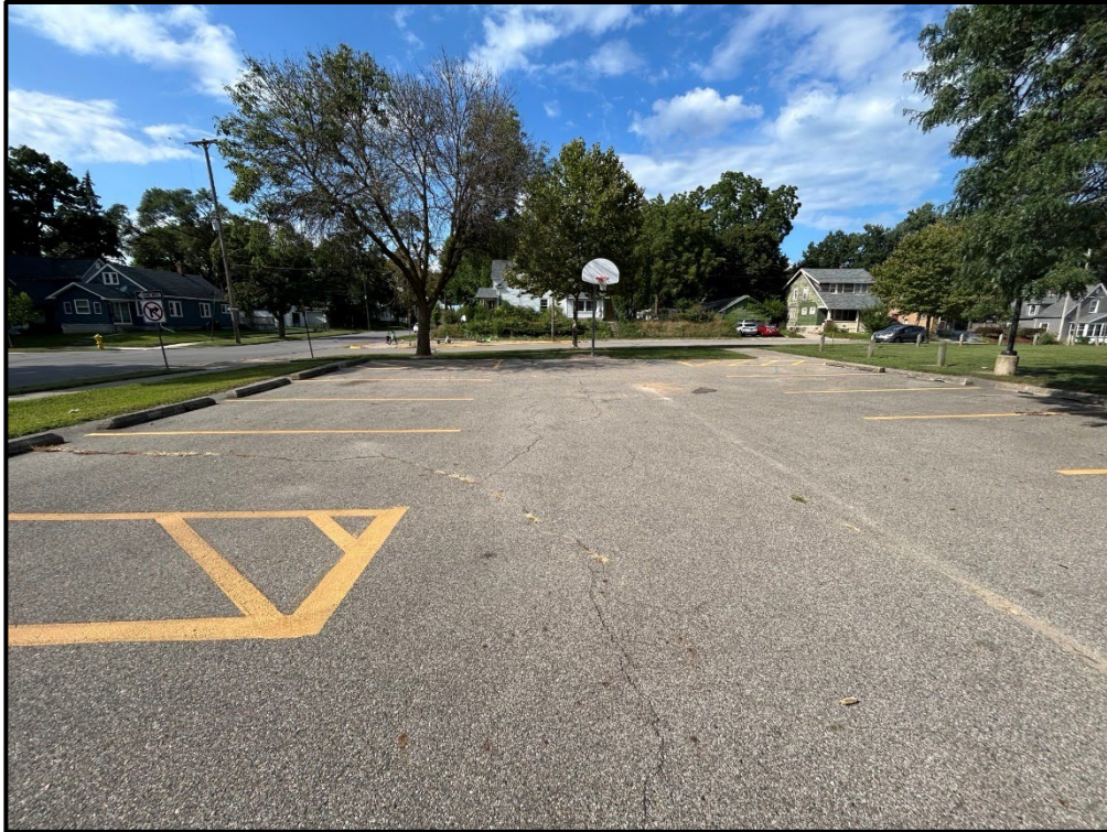
Houseman Field, northwest parking lot, looking north
